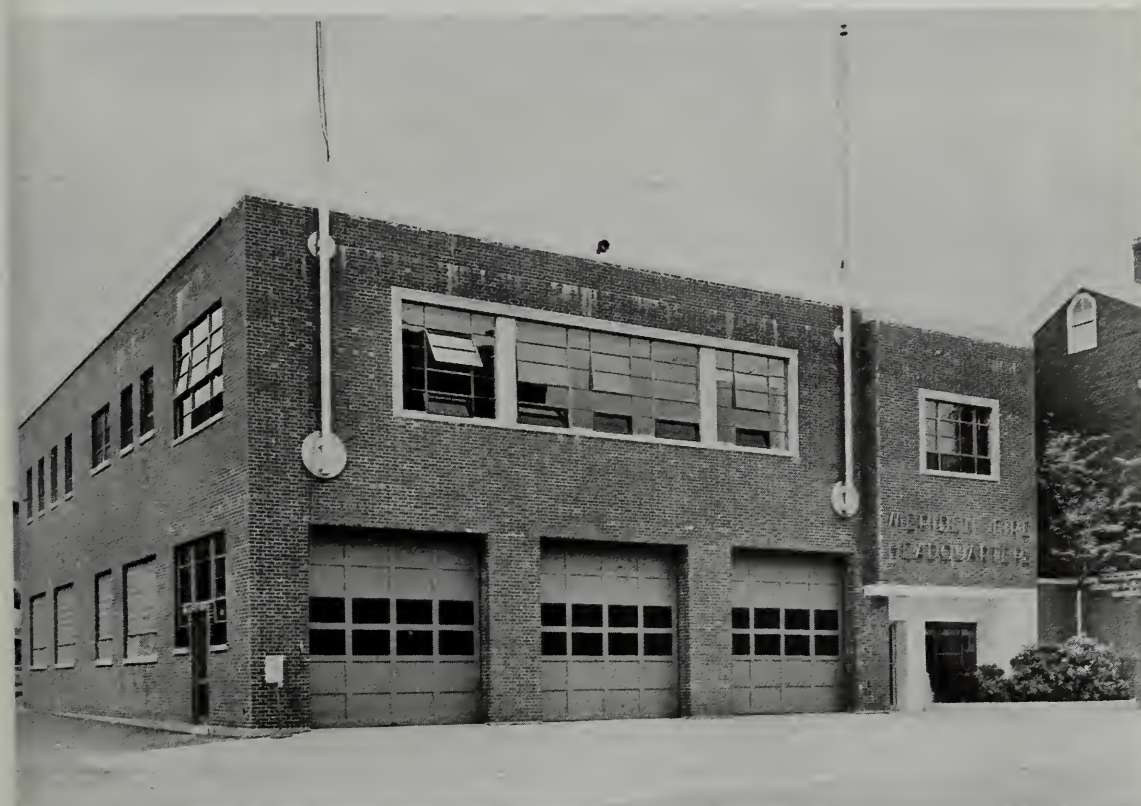
Fire Headquarters Pratt Street
